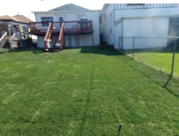
Potential exposure to contamination removed and replaced with clean soil and surface treatments such as sod or beauty bark.
